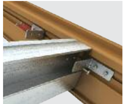
Fix rafters to ringbeam
